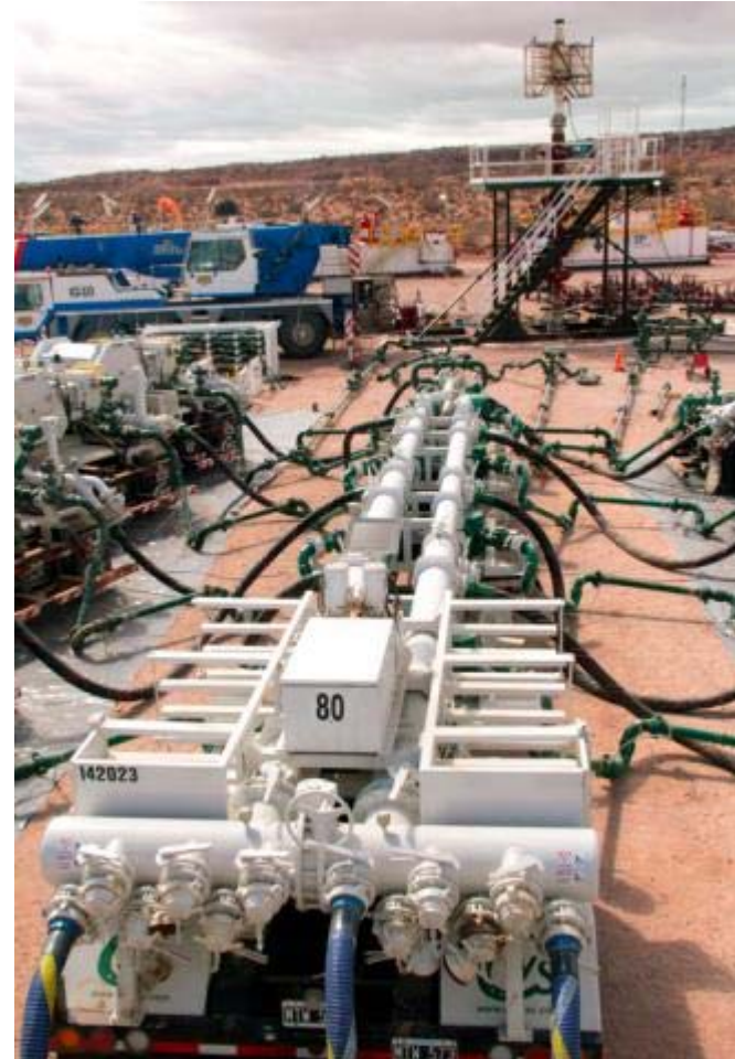
Fracturing Operation(Calfrac Photo)
